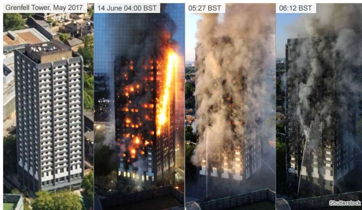
14.7.2017: Požar u Grenfell Tower-u, London
