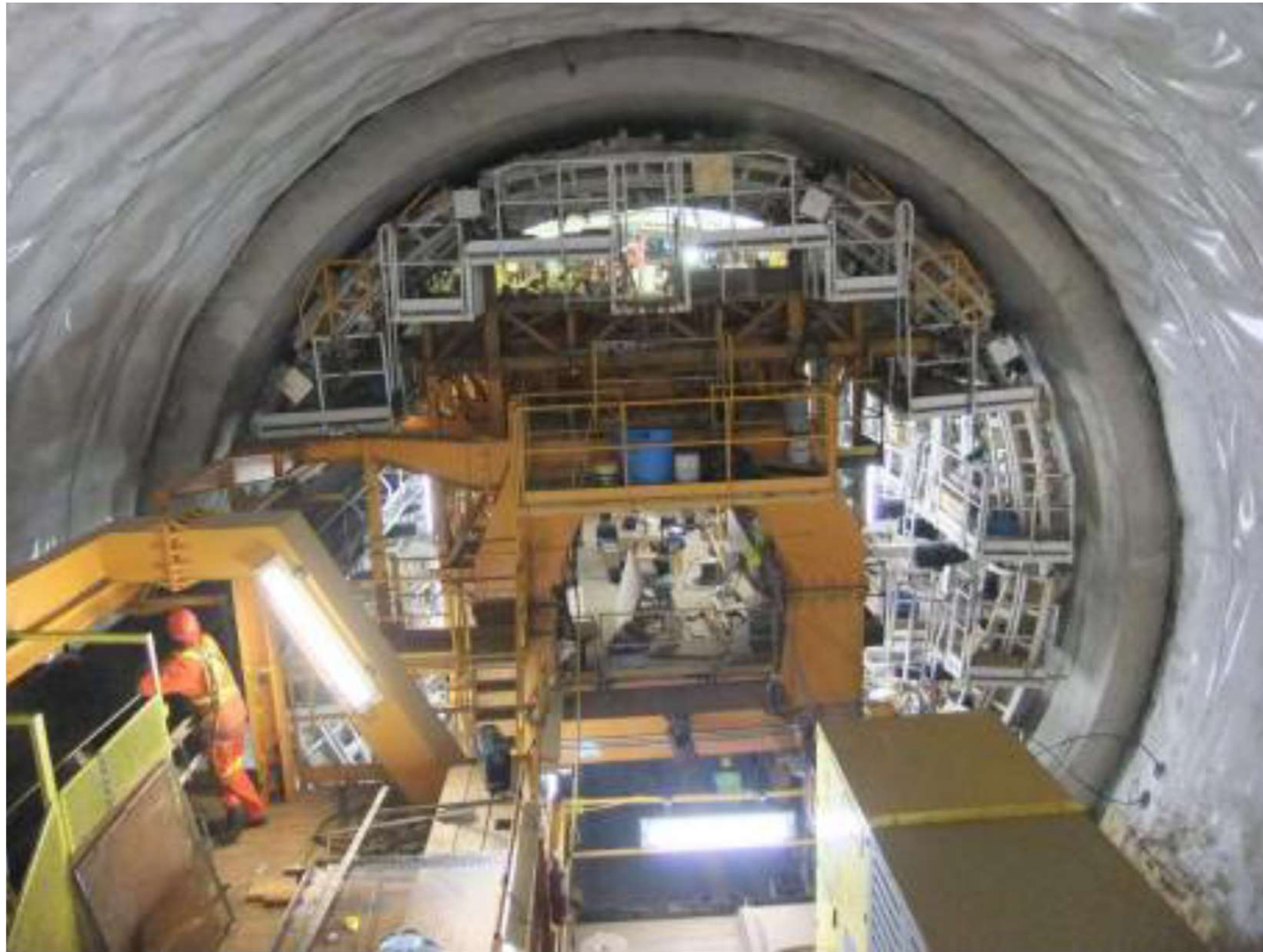
Arch Membrane and Concrete near the Outlet
