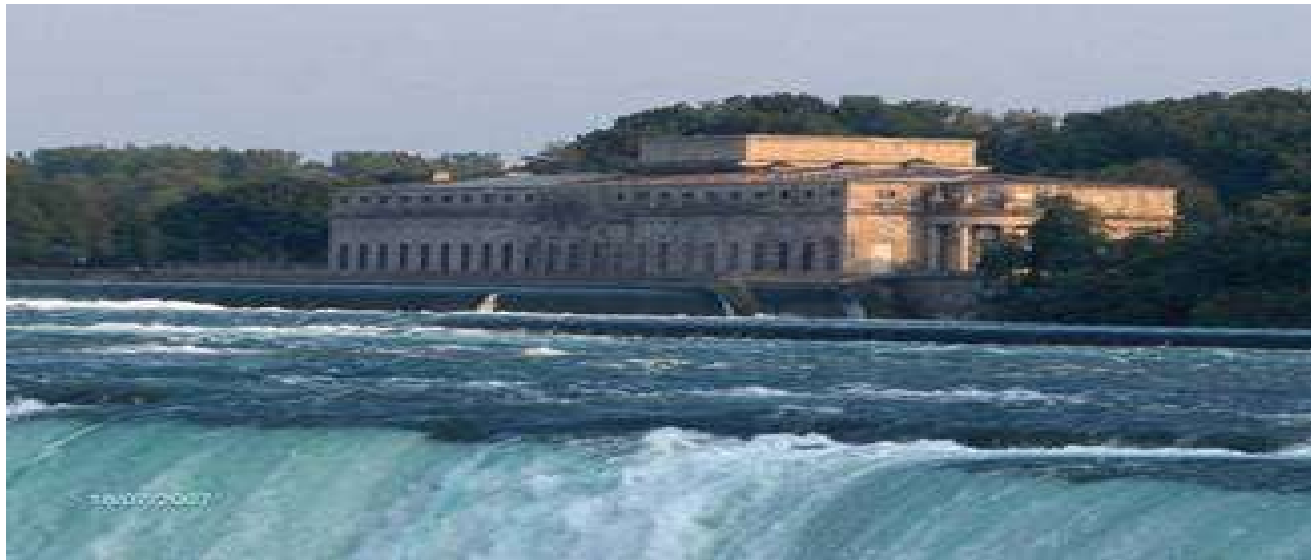
Toronto Power GS 1905 – 1974 = 120 MW (11 units)
