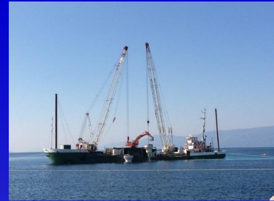
GRAVEL COLUMNS UNDER THE PIER STRUCTURE IN LAYER N1
